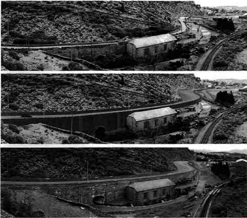
Figure 8.5 Review and monitoring: what actually happened compared with what was predicted in the LVIA
